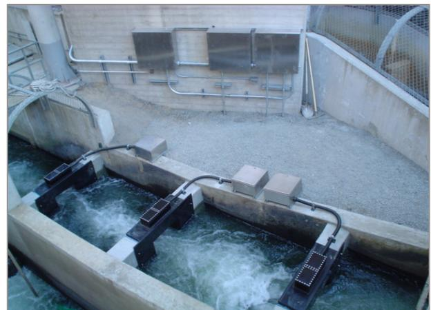
Figure 3 - There are three antennas, in adjacent weirs, in the adult ladder at Roza Dam.
