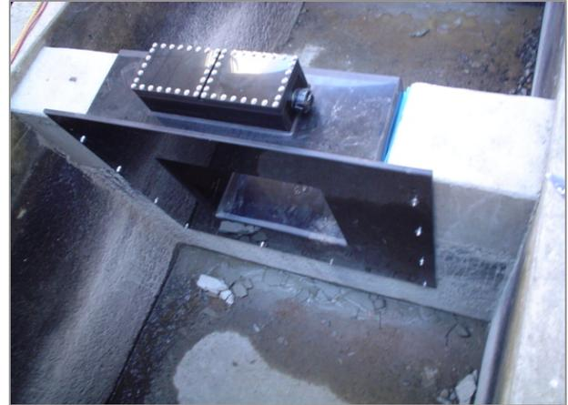
Figure 1 - A close-up of one of the PIT tag antennas installed in the fish ladder at Roza Dam.
