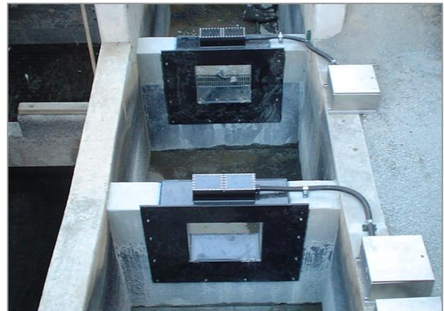
Figure 2 - All fish ascending the ladder must pass through these antennas.
