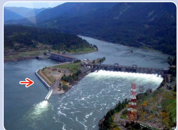
Aerial photo of Bonneville Dam taken by the U.S. Army Corps of Engineers. The arrow points to the straight section of the exit flume for the new corner-collector bypass system where the PIT-tag antennas will be installed.
