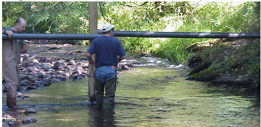
PIT Tag antenna installation at USFWS research station at Abernathy Creek.
