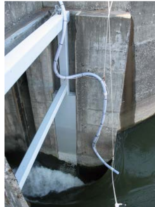
Figure 4. The left photo shows the deck where fish are held in tanks and released. The right photo shows the hose leading down to the entrance of the corner-collector flume.
